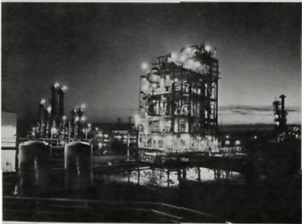
↑ An oxide reaction unit—part of Montreal East's vast chemical complex—where ethylene is converted into ethylene oxide.
